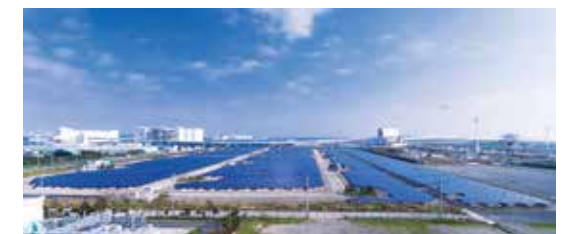
Ukishima Solar Power Plant
